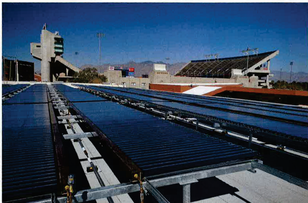
Left: Feed and inlet lines connect to the solar banks. More than 3,500 feet of Cerro copper pipe was used. Right: The unique setup allows the university to generate chilled water and pool heating from the same solar field.
